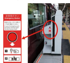
Sliding platform screen door emergency button
